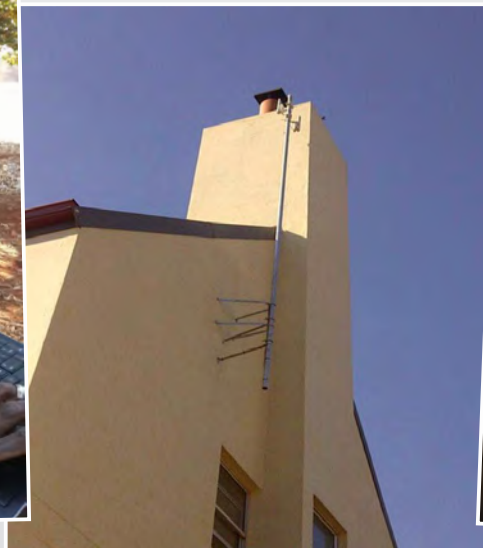
Wireless Transceiver at Control Room
