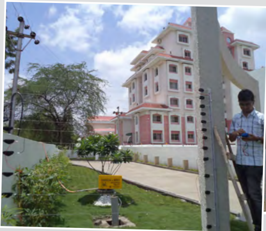
Security Fence Installation, India
