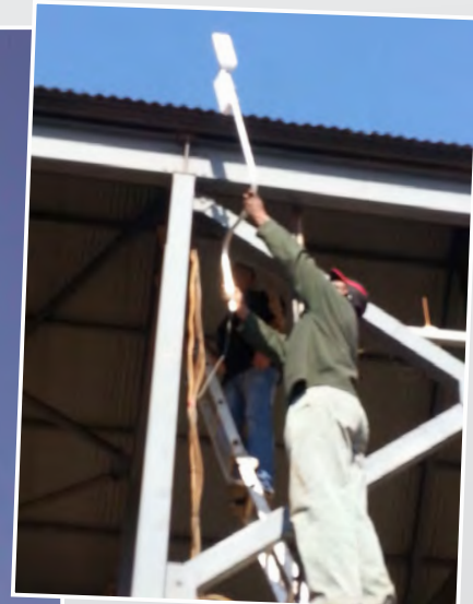
Wireless Repeater at Entrance
