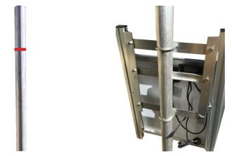
4. Loosen the 6 bolts on the inside of the frame. DO NOT completely remove these bolts. Lift the bottom of the solar panel until the attached arms holding it are angled at 90 degrees. Tighten all 6 bolts again and face the panel north.
